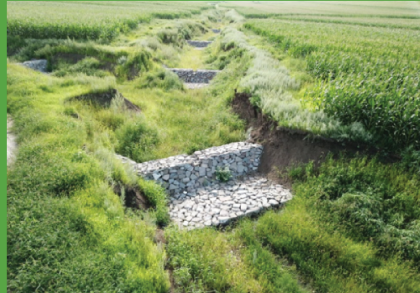
Gully control structure
